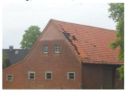
Some ceramik slates blown away on the west side of the building. Ratio <20%. DI Roofs: DoD1 (isolated tiles <20%) results in IF0+ / F0T1.
