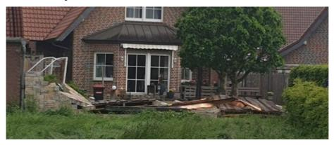
Wall collapsed. Single row brick structure. Failure point unknown.
