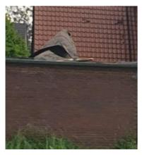
Roof cover partly lifted, but not ripped-off and thrown. According to photo material, loss ratio may reached >20% at a rough estimate.
