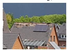
Some parts of slates blown off on the west side of the building. Damage is limited to the upper section of the roof. Loss ratio about 20-25%.
