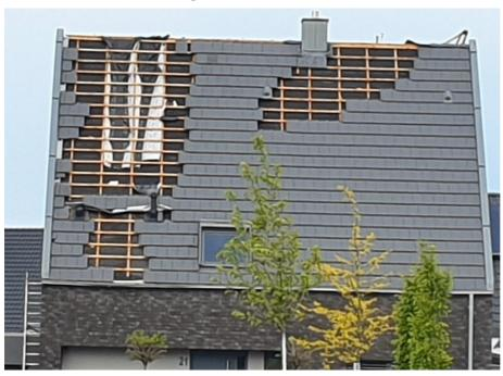
Large parts of slates blown off on the west side of the building. Loss ratio 40-50%. DI Roofs: DoD2 (20-50%) results in IF1 / F1. It is not clear whether one can expect a high-end F1 rating here or not. Damage cannot be estimated with additional T-Scale.
